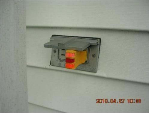
7.6 Picture 1 GFCI device failed to trip
