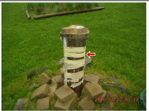
13.0 Picture 1 Masking tape holding electrical line
