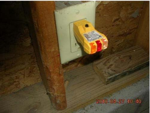
7.5 Picture 1 Incorrectly wired GFCI outlet
